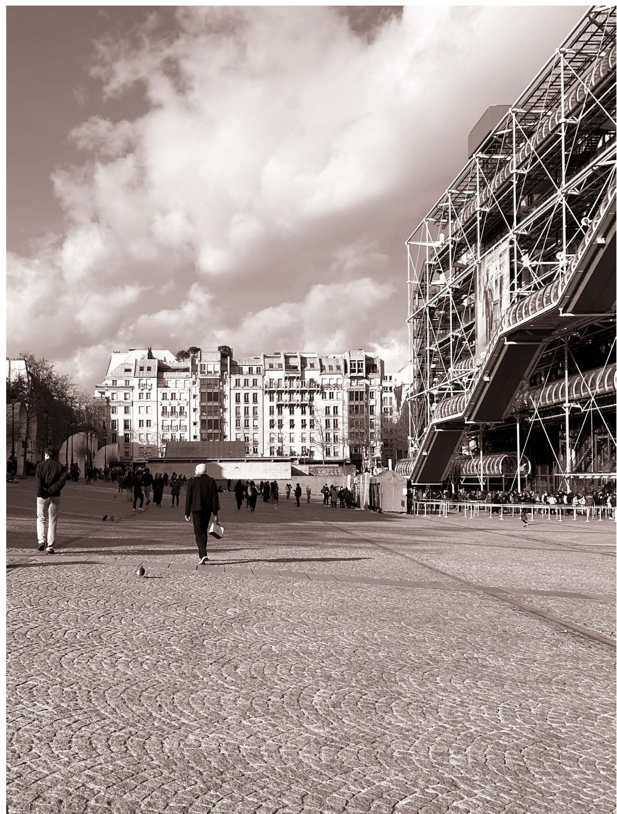
Fig. 2 Centre Pompidou, Paris, France
