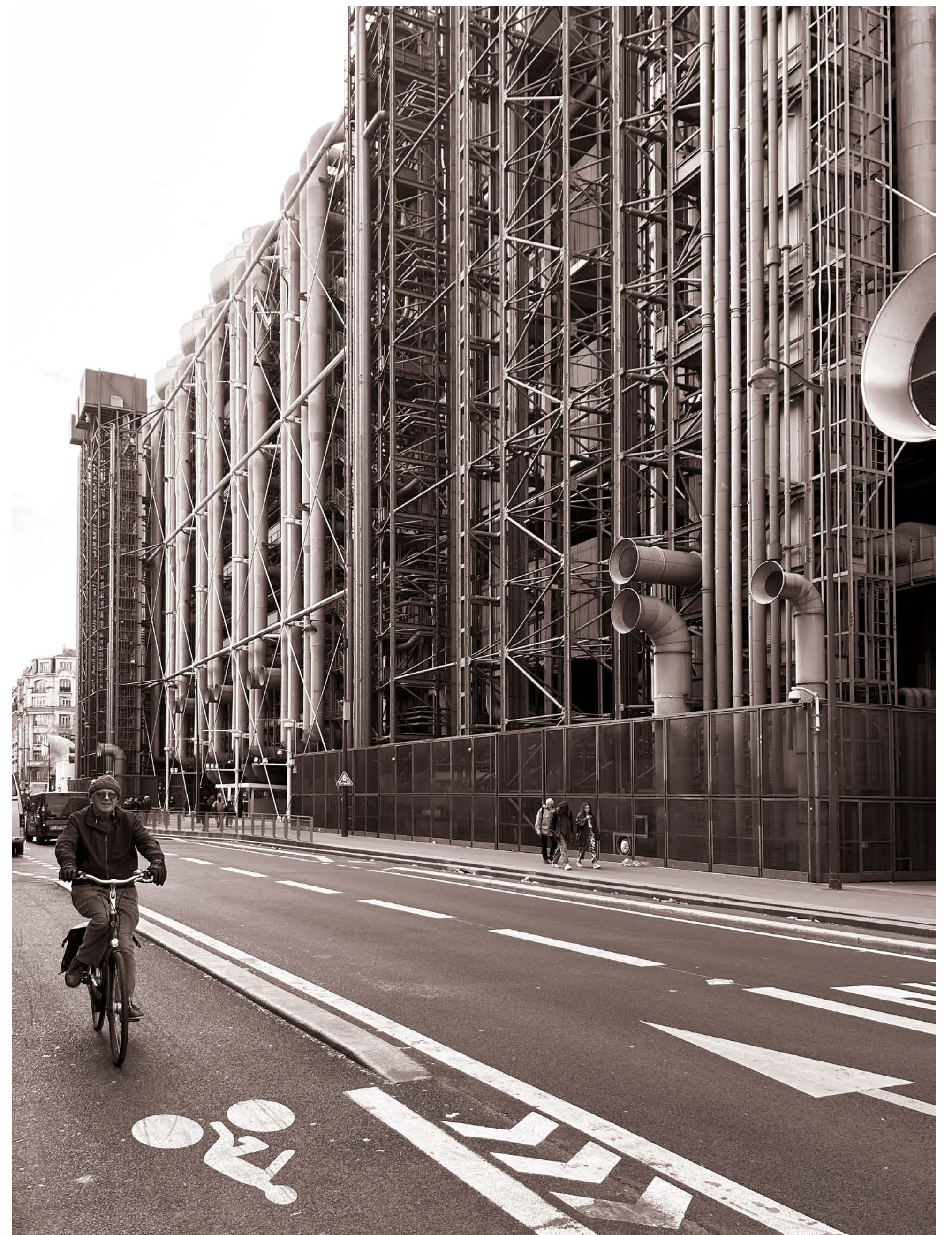
Fig. 3 Centre Pompidou, Paris, France
